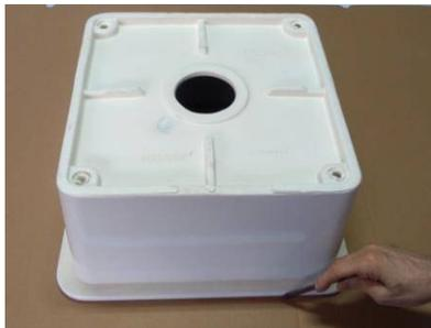
2. Draw a second line the correct distance inside the marked line based on the sink you have.
